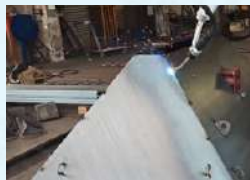
Steel Structure Weld
