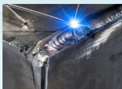
Mold Corner Repair
