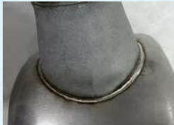
Carbon Steel Arc Weld
