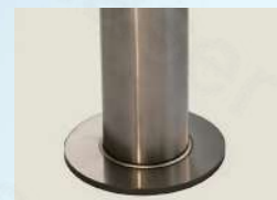
Industrial Piping Seal Weld
