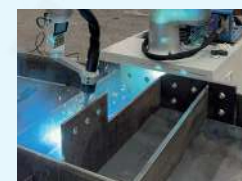
Steel Structure Weld
