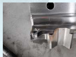
Precisely Fill the Defects
