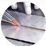
Weld Seam Cleaning
